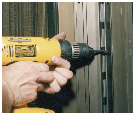
▲ Installing screw in frame leaf. Hinge is in open position, showing hinge bearings.
