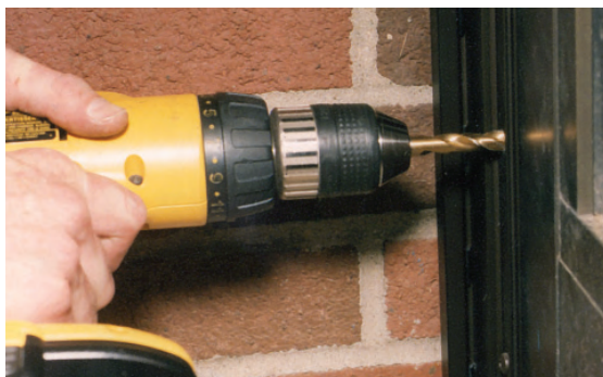
▲ Drilling fastener hole through door leaf hole into face of door.
