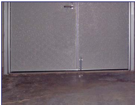
After - with Adjustable Bottom Brush
