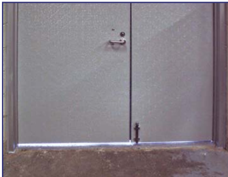
Before - without Adjustable Bottom Brush
